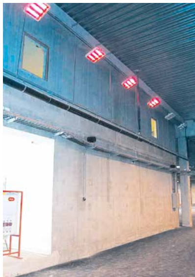
IRCF can be mounted on the wall or on the ceiling and is suitable in buildings which are used sporadically like this go-cart track starting area.
